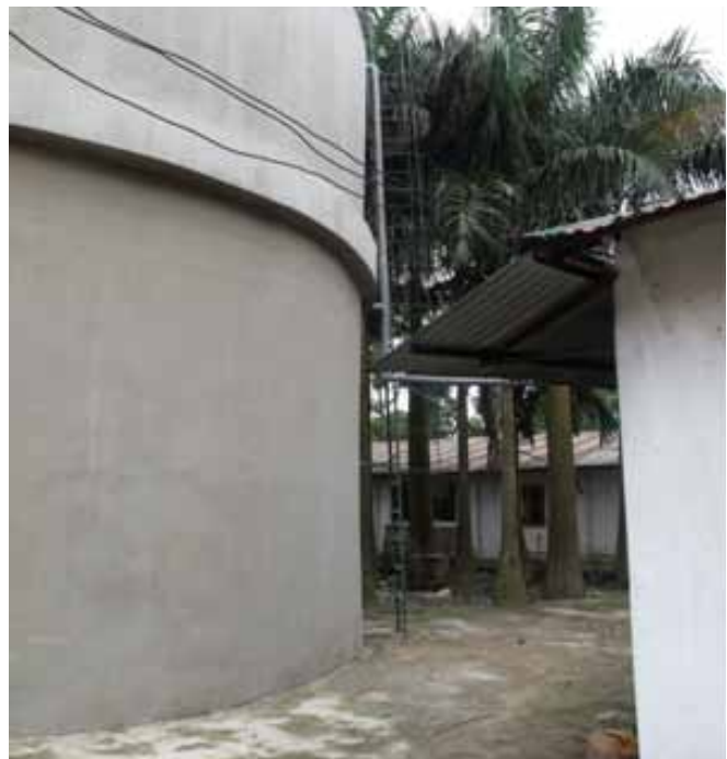
Biogas plant (Photo courtesy: Le Thi Xuan Thu)
