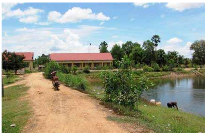
Commune building to have solar panels installed.
