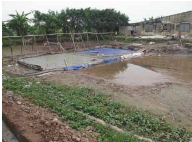
Project location, Nam Binh province: Initial works
