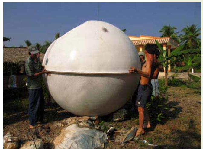
Shaping a household biogas digester at a project site
