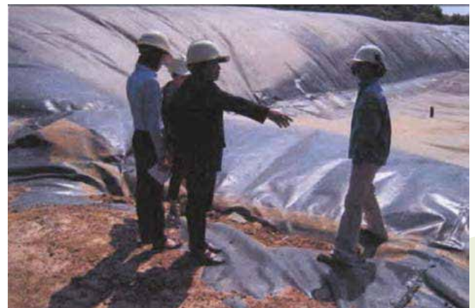
Foreign experts discussing Covered Lagoon Bio-Reactor (CLBR) technology in TBEC Kalasin plant
